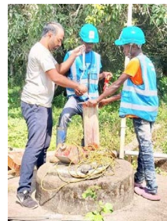
Final touches are being made to
