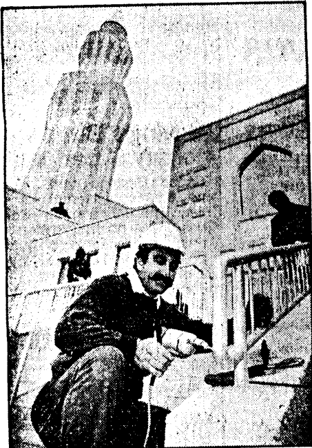
RIVETING WORK: Mohammad Ashraf Nazer puts finishing touches to main entrance of the mosque.
