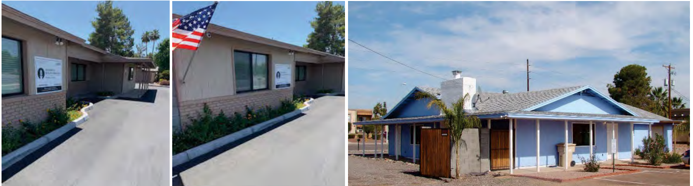
Front views of Bait-ul-Amn (left). Back view from southwest.
