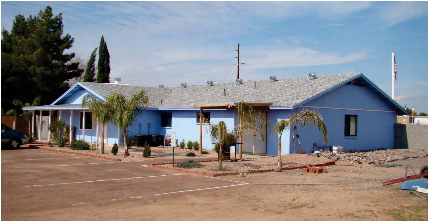
Bait-ul-Amn, back view from southeast.
