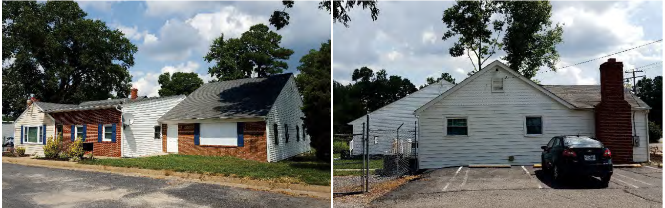
Left: View from the west. Right: View from the north.
