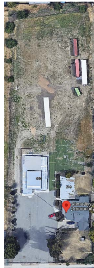
At the bottom right is the missionary residence. At the bottom left are meeting halls, kitchen and dining areas.
