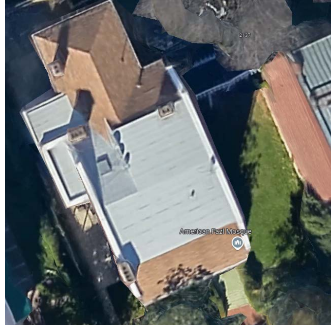
An aerial view of the site.
