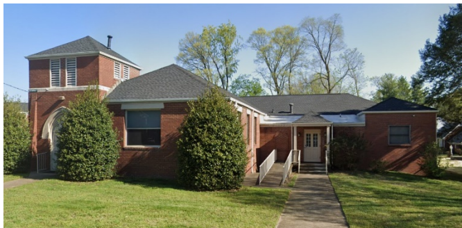
View from south of the building. [Google]
