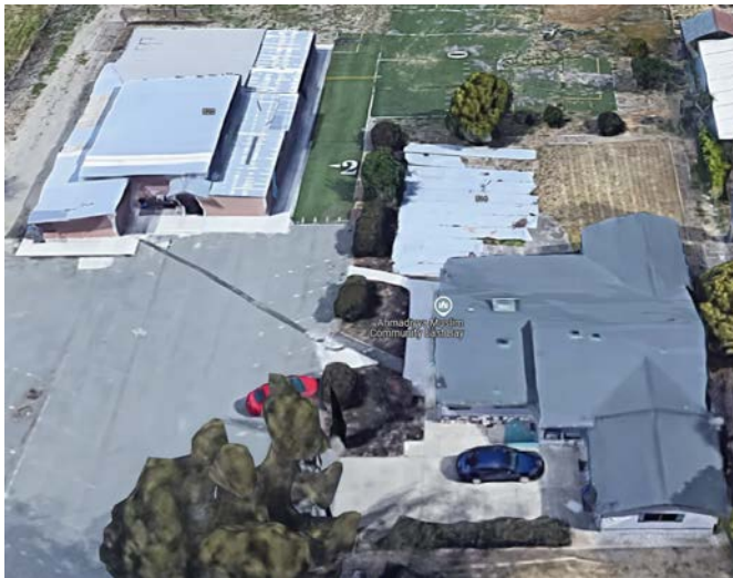
To the left are meeting halls, kitchen and dining areas. To the right is the missionary residence.
