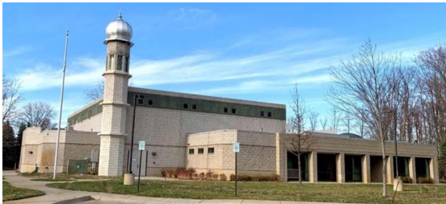
Back view of the complex. To the right are offices and to the left are a kitchen and a large arena to cater events.
