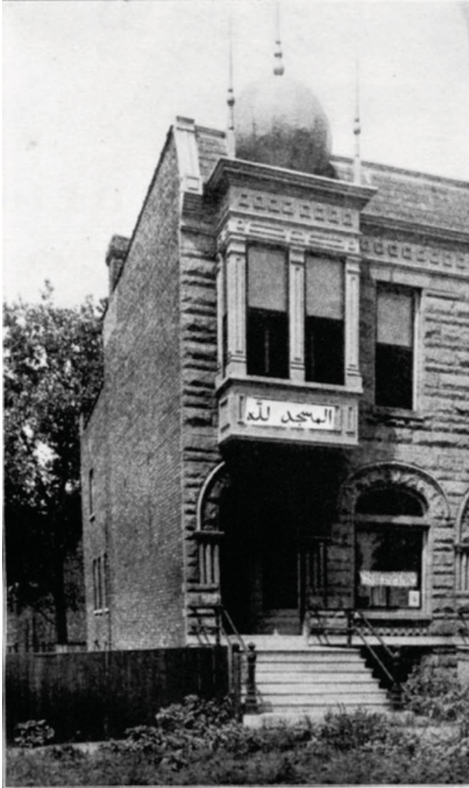
Building purchased in Chicago and converted to a mosque and a mission house.
