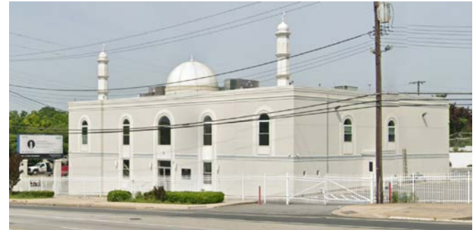
A view of the mosque from the southeast. [Google]
