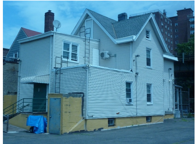
View from the southwest.
