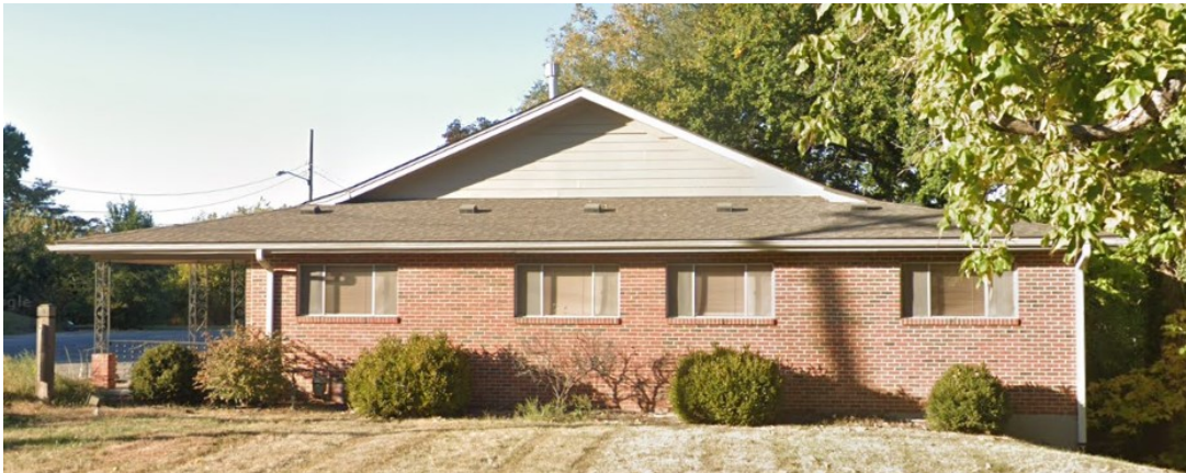
View of the building from the south.
