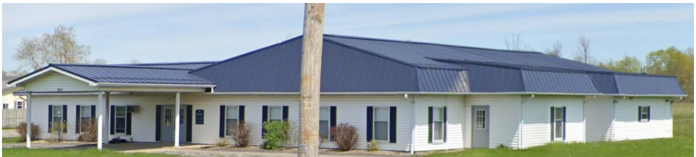
View from the southwest. (Google) ★
