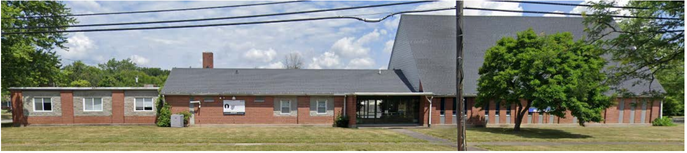
View from south. [Google]
