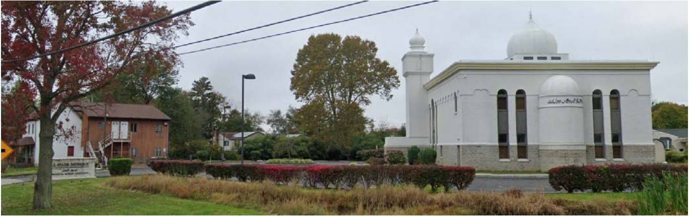
Front view of the Al-Nasr Mosque
