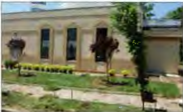
New mosque under construction in St. Louis, Missouri.
